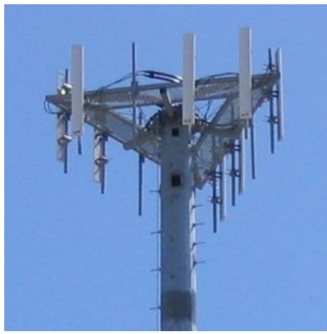
A typical base station (Source: Wikipedia ( https://en.wikipedia.org/wiki/Sector_antenna ))
